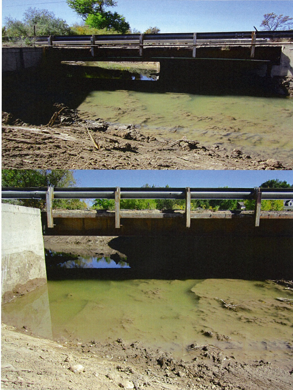
26 Road Bridge Opening – After the Cleaning in the Fall of 2011
