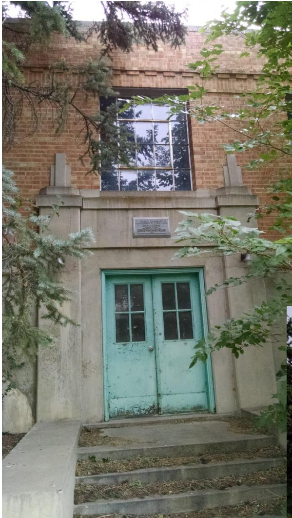
North Façade Entry Name/Date Panel
