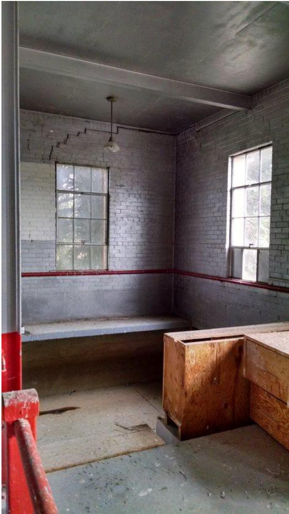
Interior – Northeast Corner
