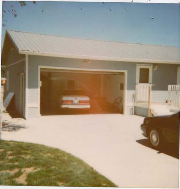
Front-South side Picture (A)
