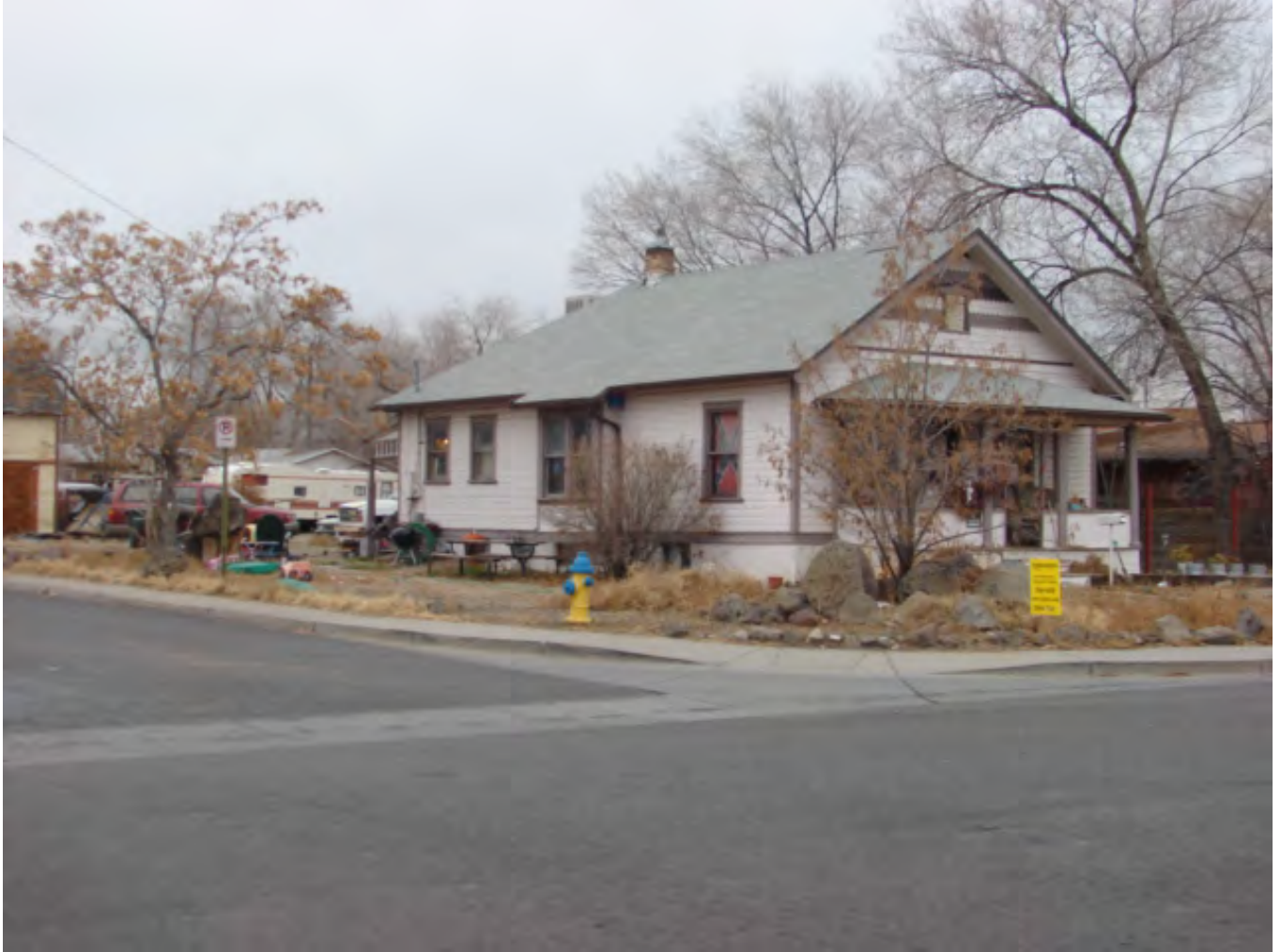
Photo 1 - 1213 N. 15th St. looking from SE
