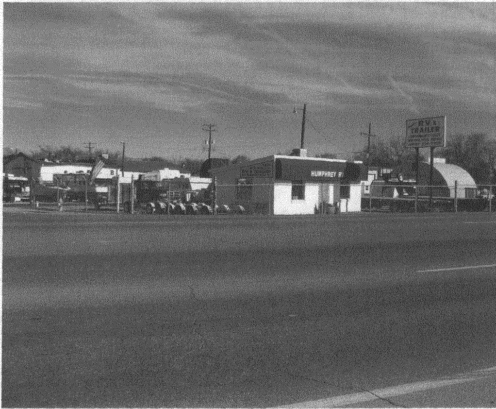
VIEW TO THE NORTHEAST OF SOUTHWEST CORNER OF SITE AND OFFICE BUILDING
