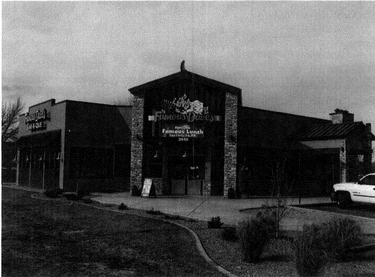
Photograph #1 – Front view of building located at 2440 Highway 6 & 50
