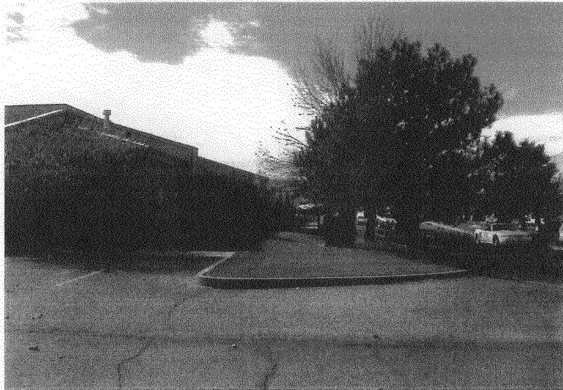
West side of existing building (to be demolished). Photo taken Oct. 24, 2006
