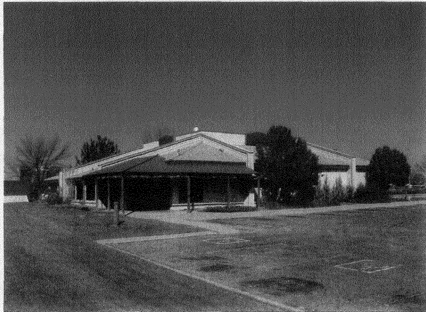
South-east side of existing building. Photo taken Oct. 24, 2006
