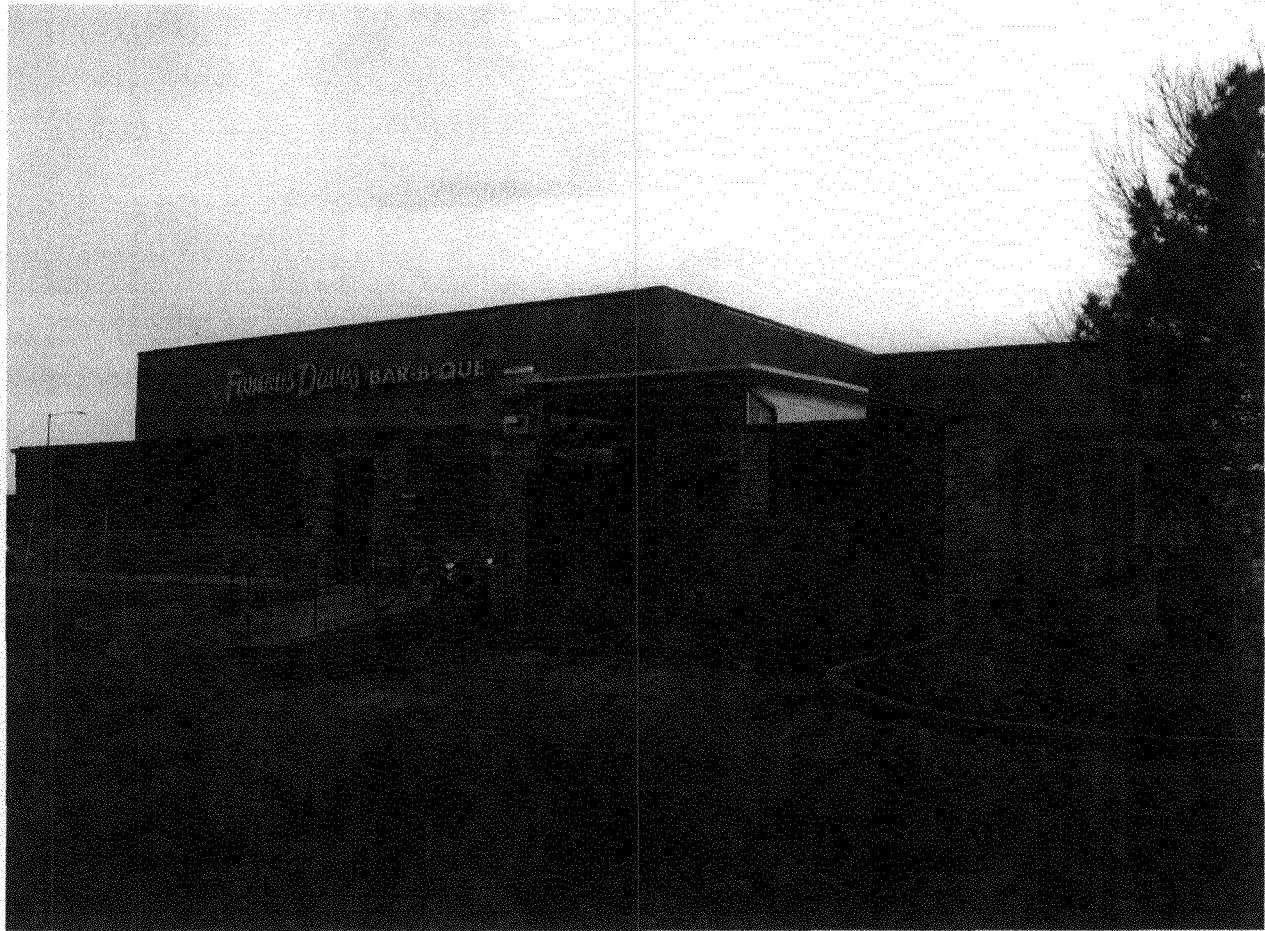
Photograph #2 – Rear view of building located at 2440 Highway 6 & 50
