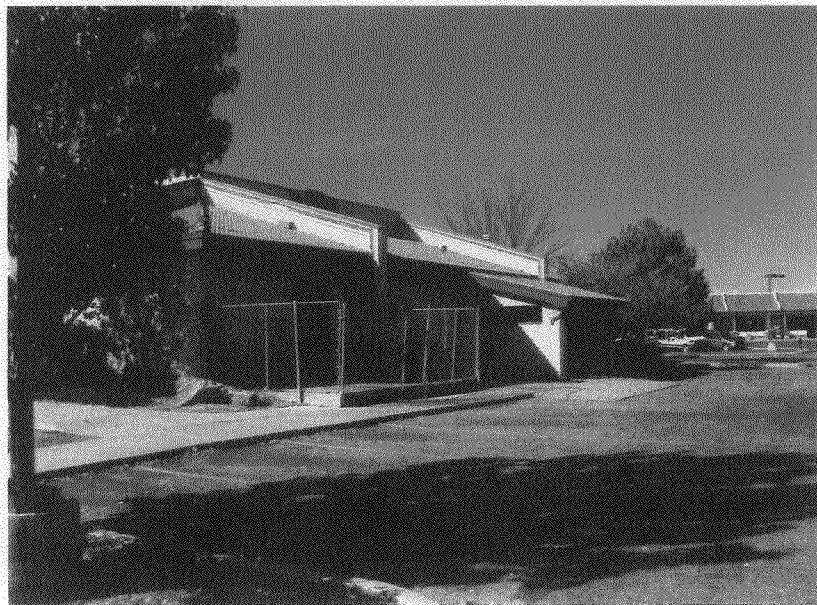
South side of existing building. Photo taken Oct. 24, 2006
