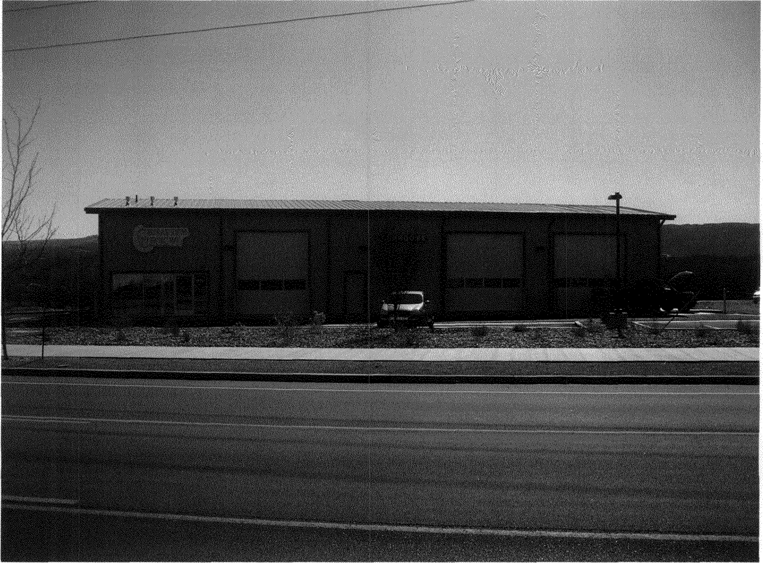
Front view taken March 10, 2009
