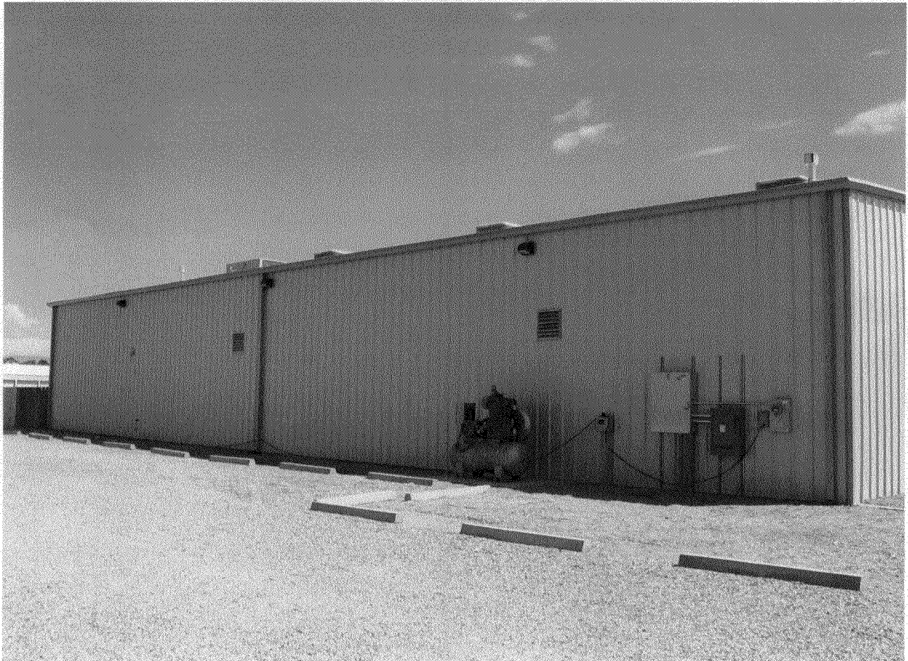
Photograph #2 – Rear view of building located at 2381-1/2 River Road, Building C
