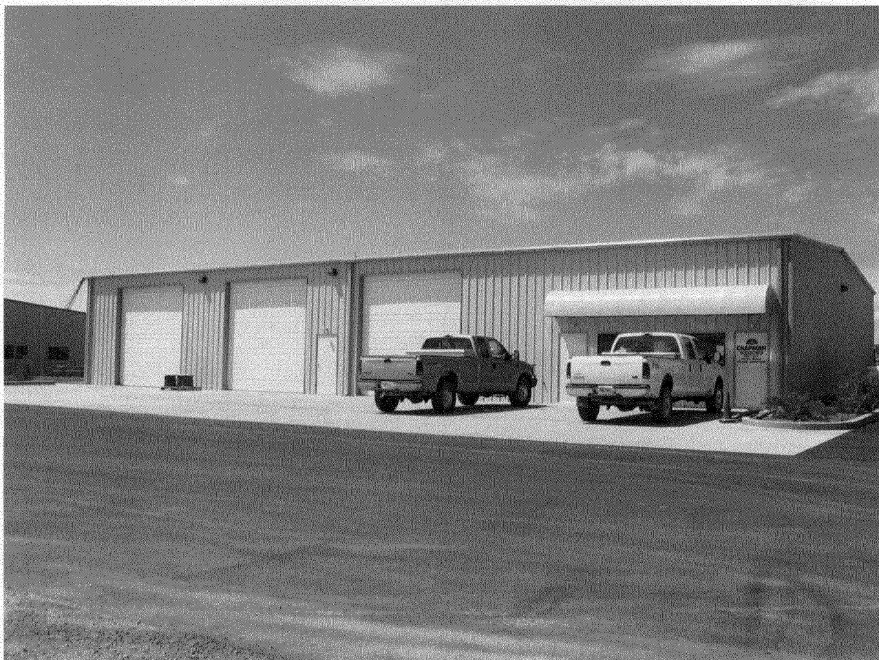
Photograph #1 – Front view of building located at 2381-1/2 River Road, Building C
