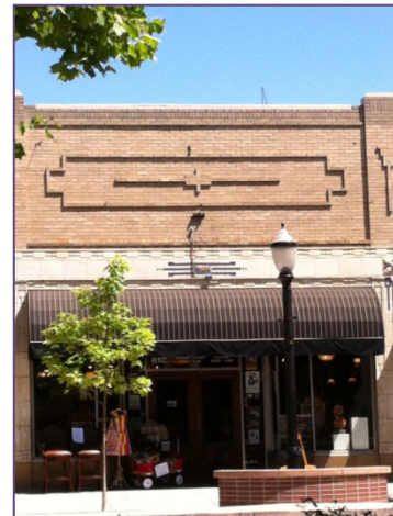
Existing Canopy on Main Street Building
