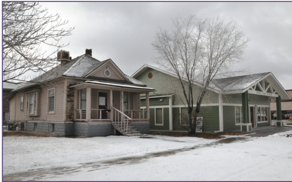
New Infill Development Building on Right
