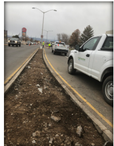
North Ave. Median Work
