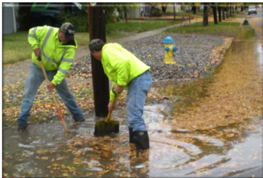
Storm Drain Cleanup
