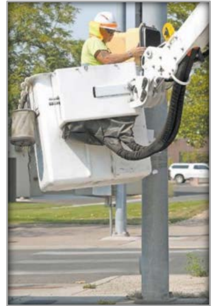
Street Light Repairs
