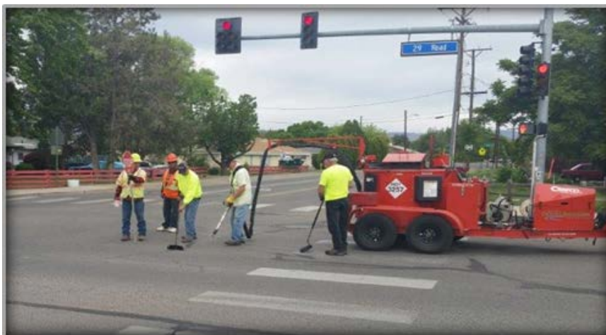
Crack Fill Operations
