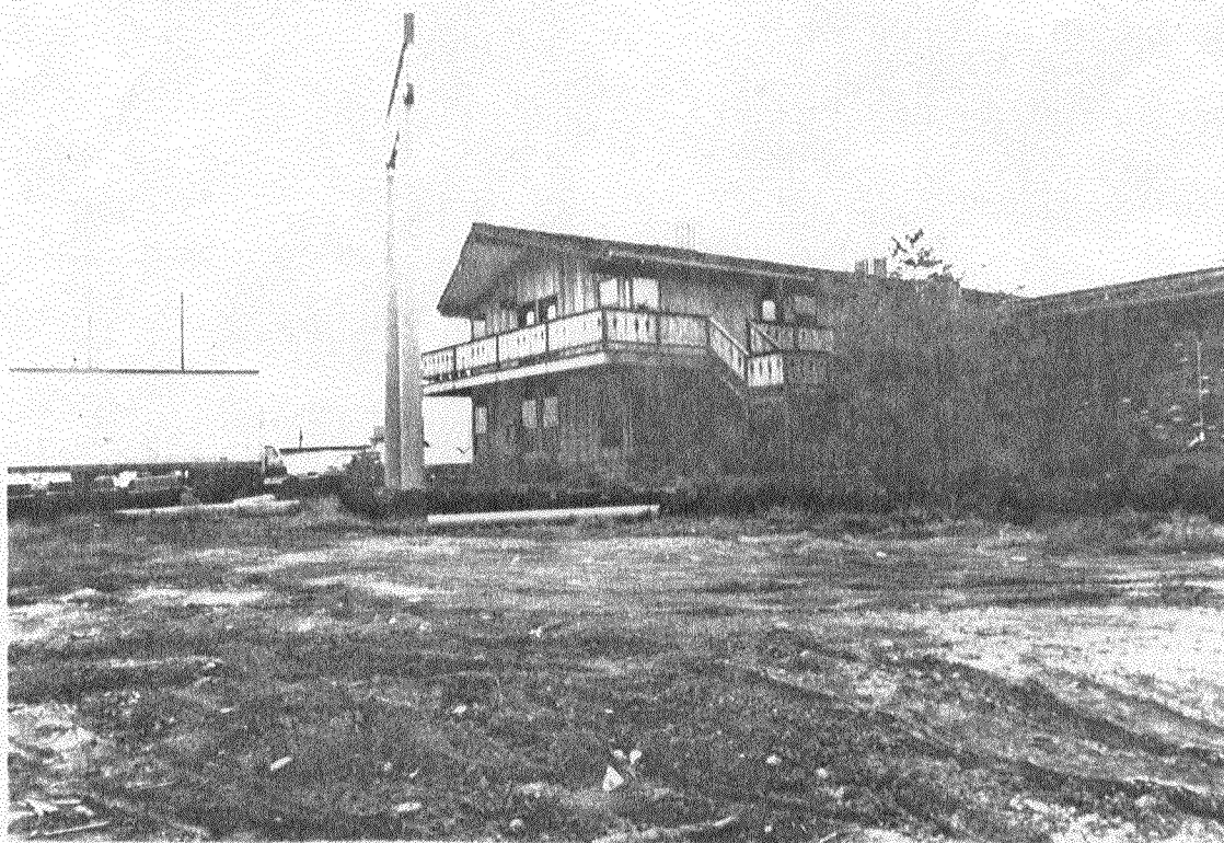
Rear of North Wing
