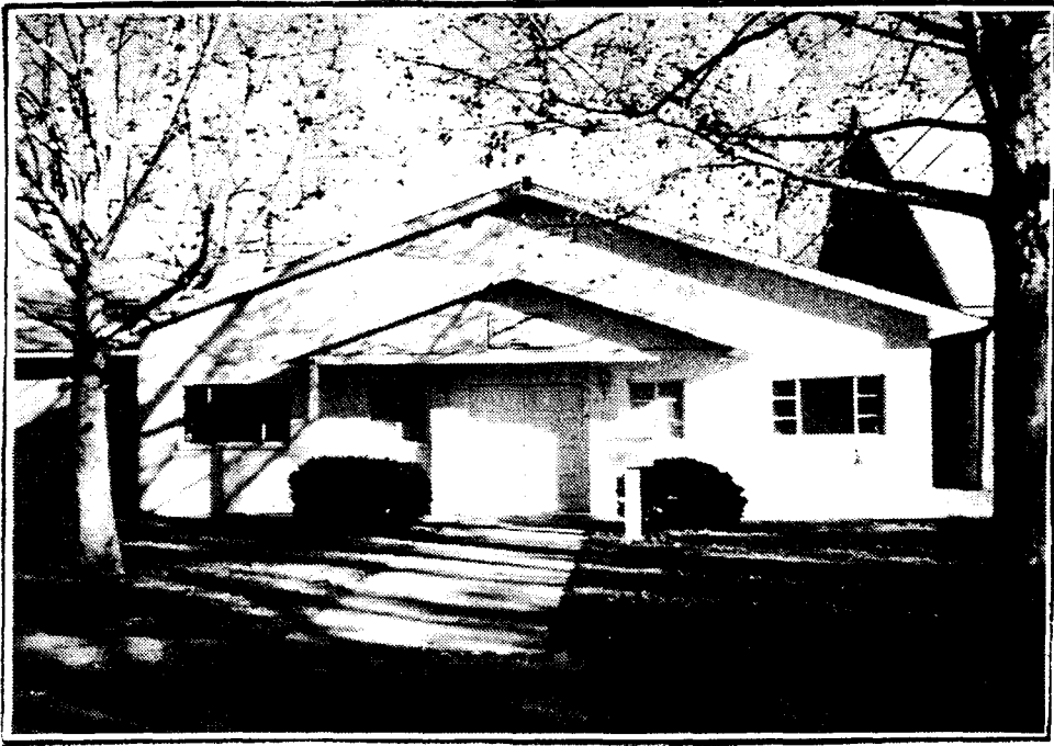
ENTRANCE TO BUILDING ON 17th STREET
