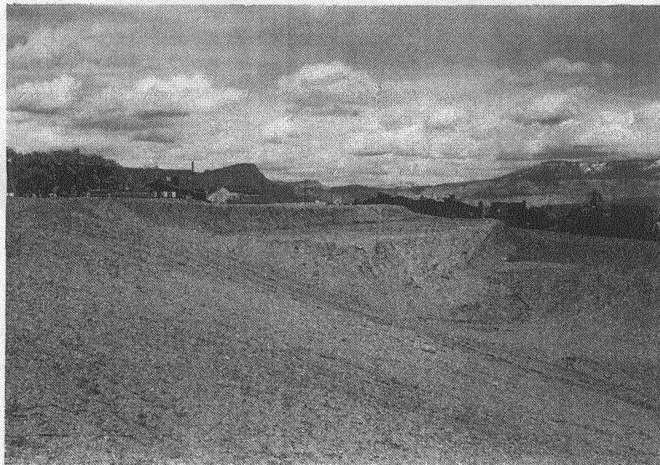
Looking northeast at the two berms on the southern portion of the site. The berms are partly in-place shale and partly man-made fill.
