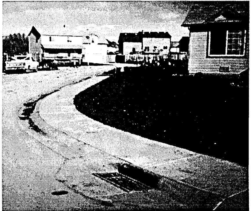
EXISTING CURB INLET ON THE WEST SIDE OF CORRAL DRIVE
