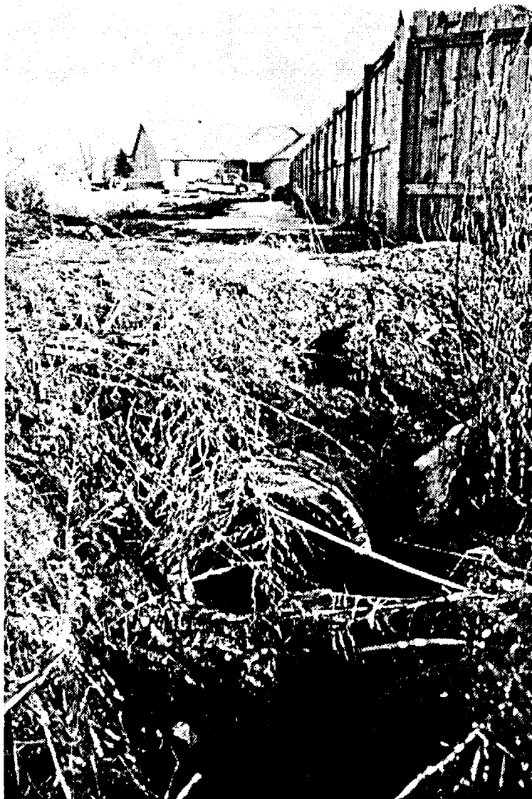
DRAIN OUTLET TO THE CLICK WASTE WATER DITCH
