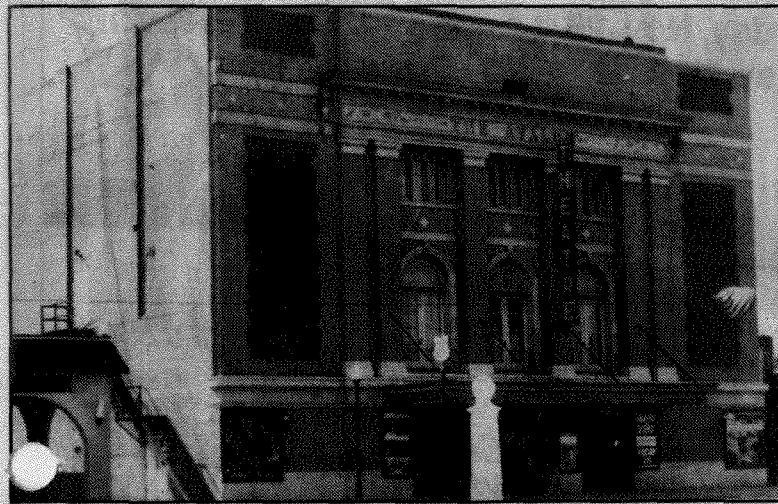
When the facade is restored, the Avalon Theatre, 535 Main St., will once again sport its 1920s look.
