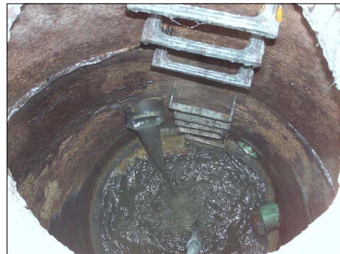
PHOTO C PEPSI LIFT STATION WETWELL TO BE REMOVED 3' BELOW GRADE & BACKFILLED
