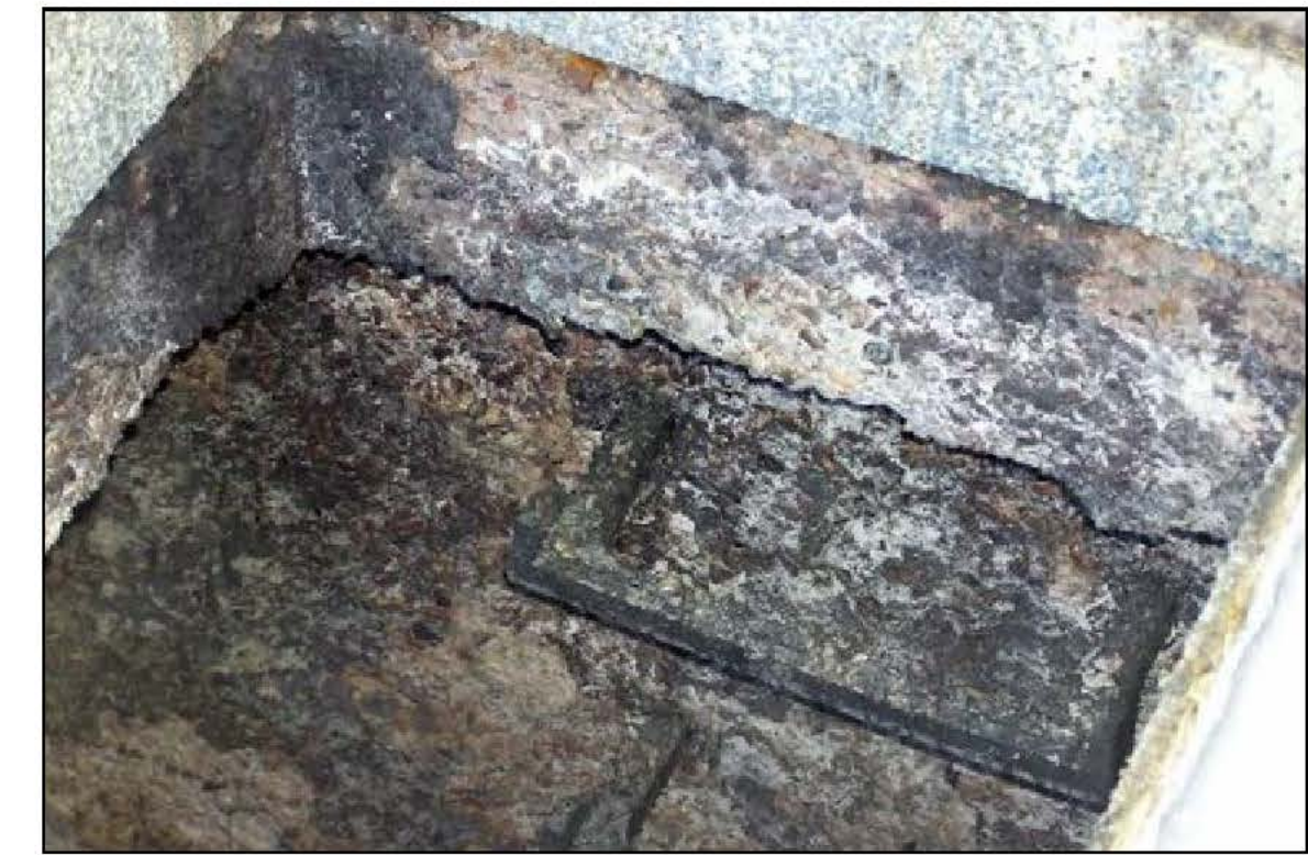
14 LOOKING SOUTH INSIDE INFLUENT CHAMBER AT SOUTH WALL AND ACCESS RUNGS
