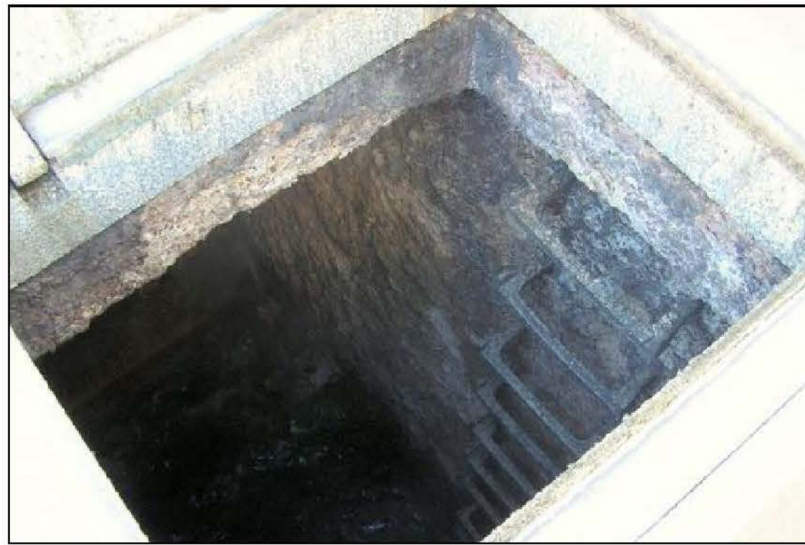
11 LOOKING SOUTHEAST INSIDE INFLUENT CHAMBER AT SOUTH WALL AND ACCESS RUNGS
