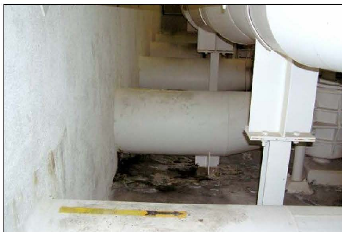
22 LOOKING EAST ACROSS PUMP ROOM AT 24" DUCTILE IRON DISCHARGE PIPES THAT PENETRATE THE SOUTH WALL OF WET WELLS 1 AND 2
