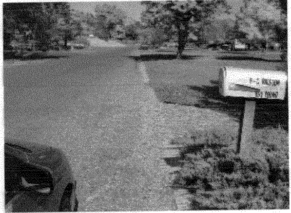
652 Young Street "gutter."
