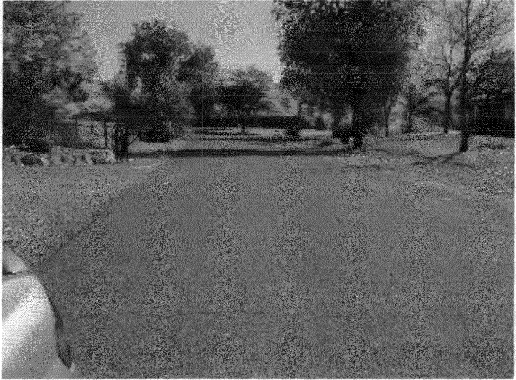
Young Court looking east.
