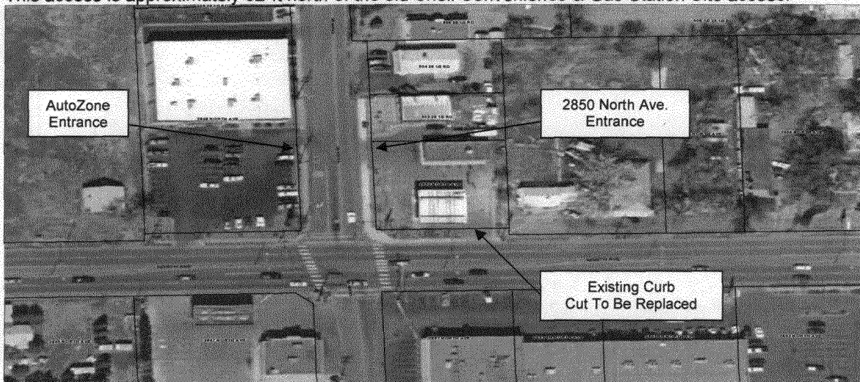
EXISTING 2850 NORTH AVENUE SITE
