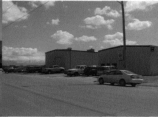
Buildings/Parking South of CAPCO
