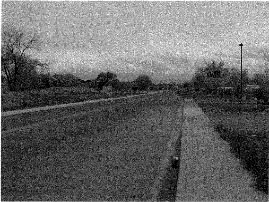
View looking north along east side of 25 \frac{1}{2} Road
