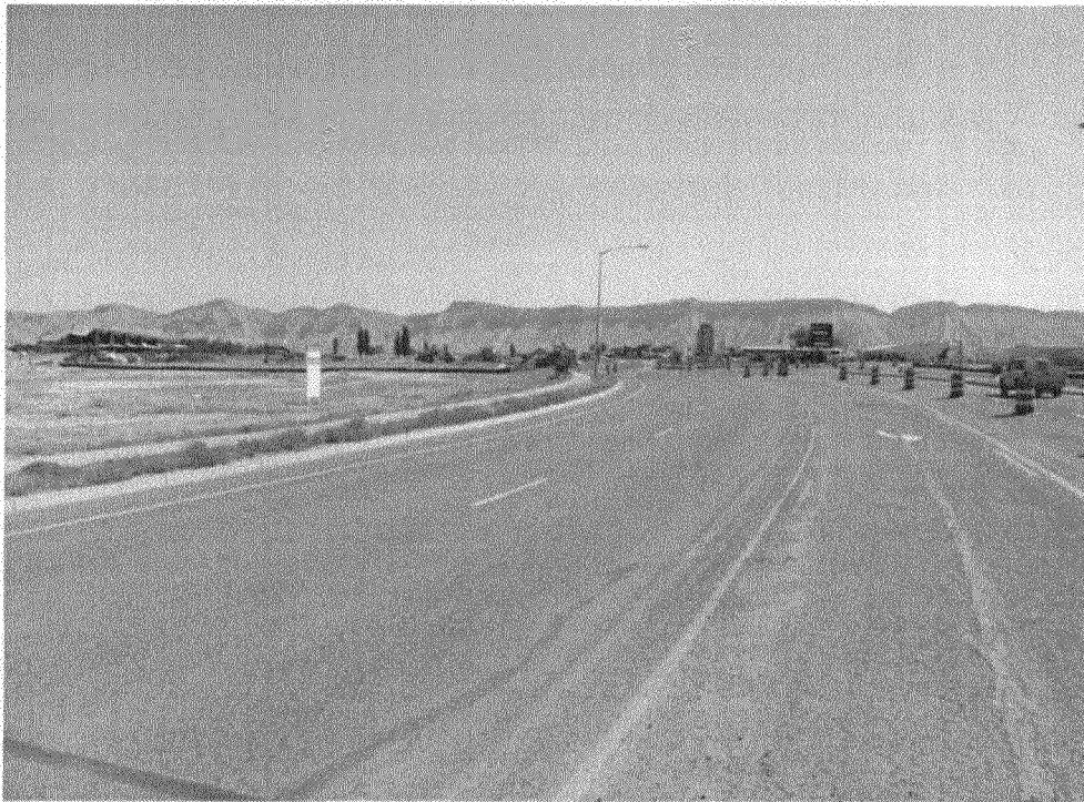
Photo #1: Horizon Drive access location (on immediate left) facing northeast..
