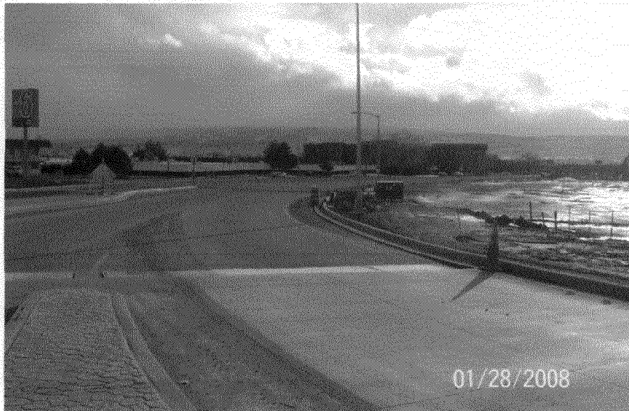
Photo 1: Looking S. down Horizon Drive (Hyatt site on right past transformer)
