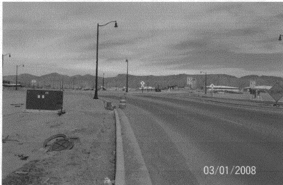
Photo 3: Looking at roundabout from north driveway location
