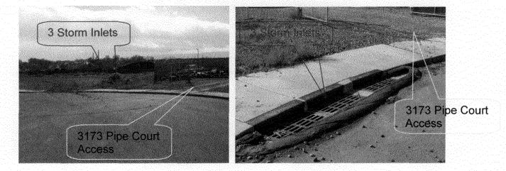
The actual "available" frontage for this access at the curb line is therefore reduced to approximately 32-ft. Per the City of Grand Junction standards for a driveway access (C-08), we must provide a five-foot curb taper transition at each side of the access which further reduces the maximum actual "driveway" width to 22-ft.
