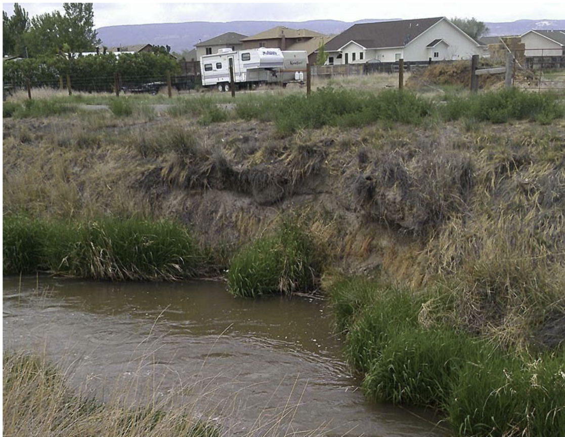
Figure 2-3 Lewis Wash Channel with Eroded Banks Pre-Construction
