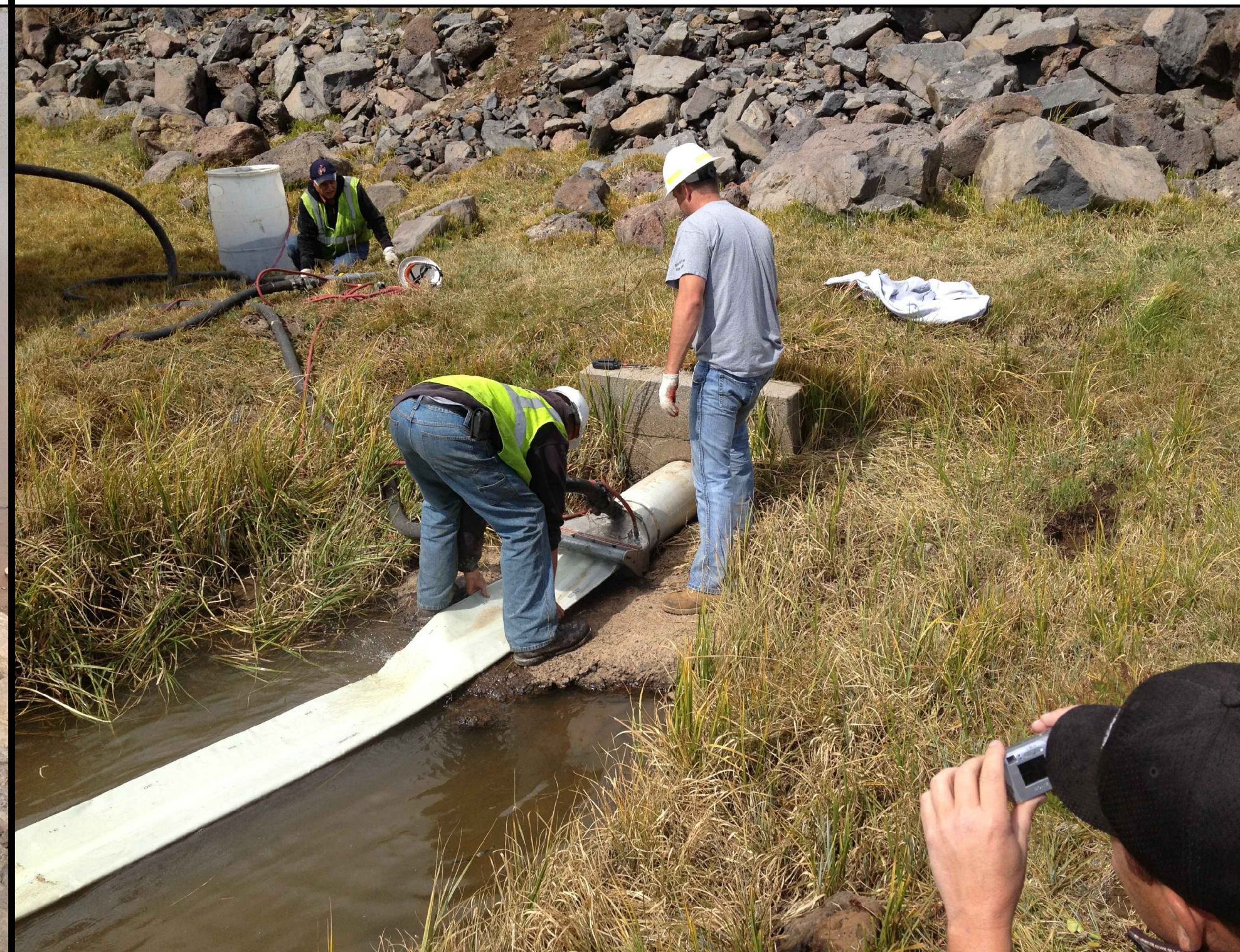
PHOTO 4: INNER PORTION OF 2 PART LINER FROM OUTLET SIDE OF DAM PUSHED AND INVERTED BACK THROUGH THE OUTER PORTION OF LINER WITH COMPRESSED AIR VIA A PIPE LINER AIR INVERSION TOOL
