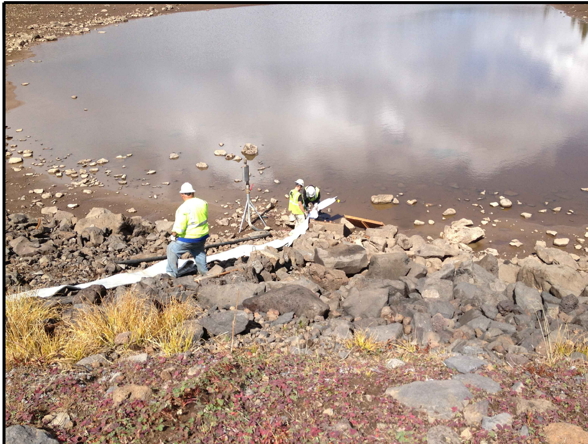
PHOTO 1: WORKERS PREPPING OUTER PORTION OF 2 PART LINER TO PULL THROUGH HOST PIPE FROM THE RESERVOIR OR INLET STRUCTURE END OF THE HOST PIPE.
