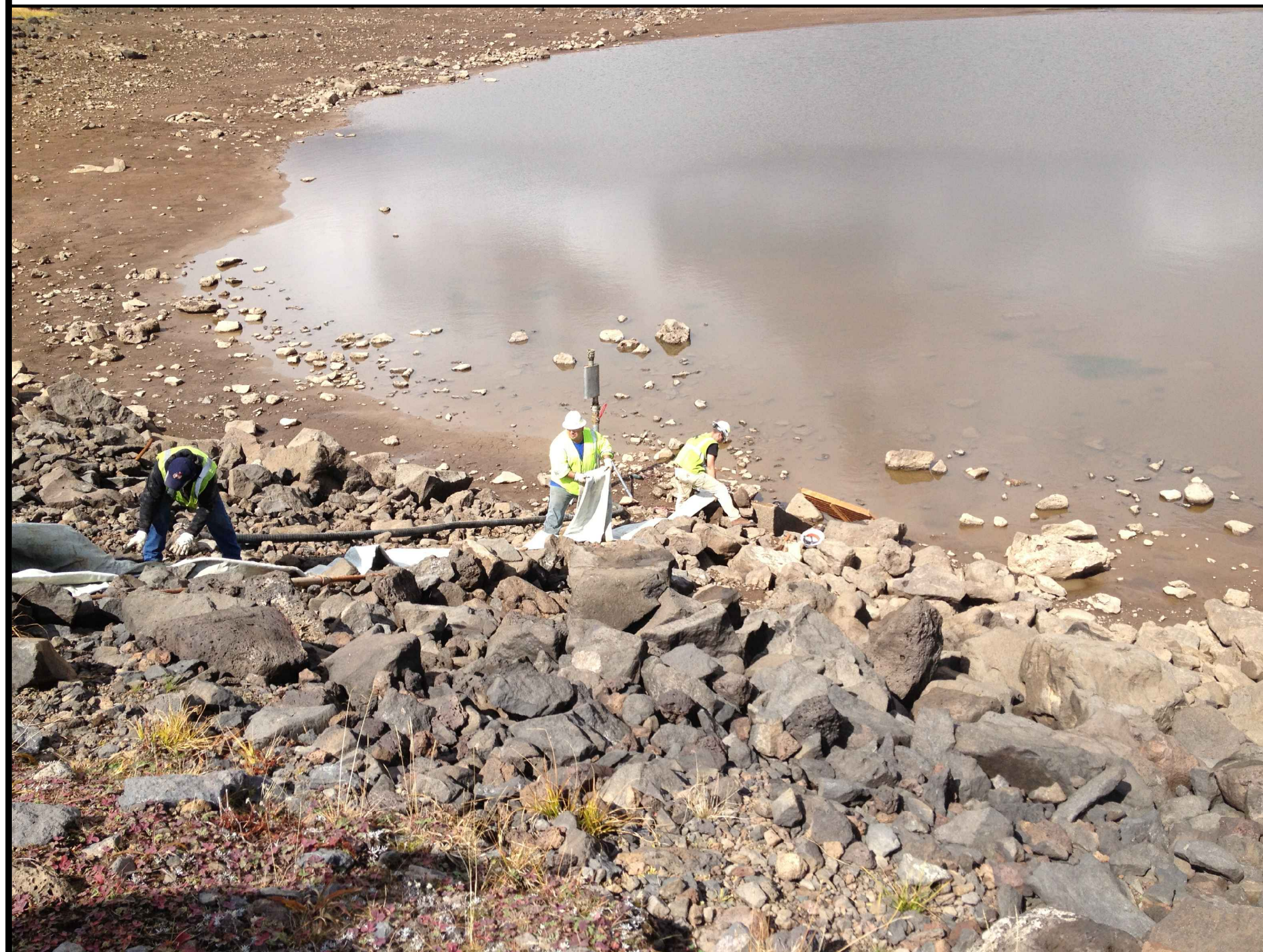
PHOTO 2: OUTER PORTION OF 2 PART LINER BEING FED THROUGH HOST PIPE FROM THE RESERVOIR OR INLET STRUCTURE END OF THE HOST PIPE AND PULLED FROM THE OUTLET END OF THE PIPE (NOT SHOWN).
