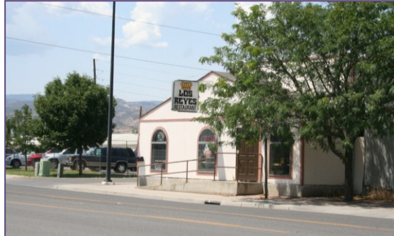
Existing Business on South 7 th Street
