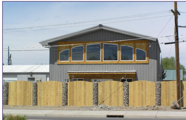
Screening Example on Riverside Parkway
