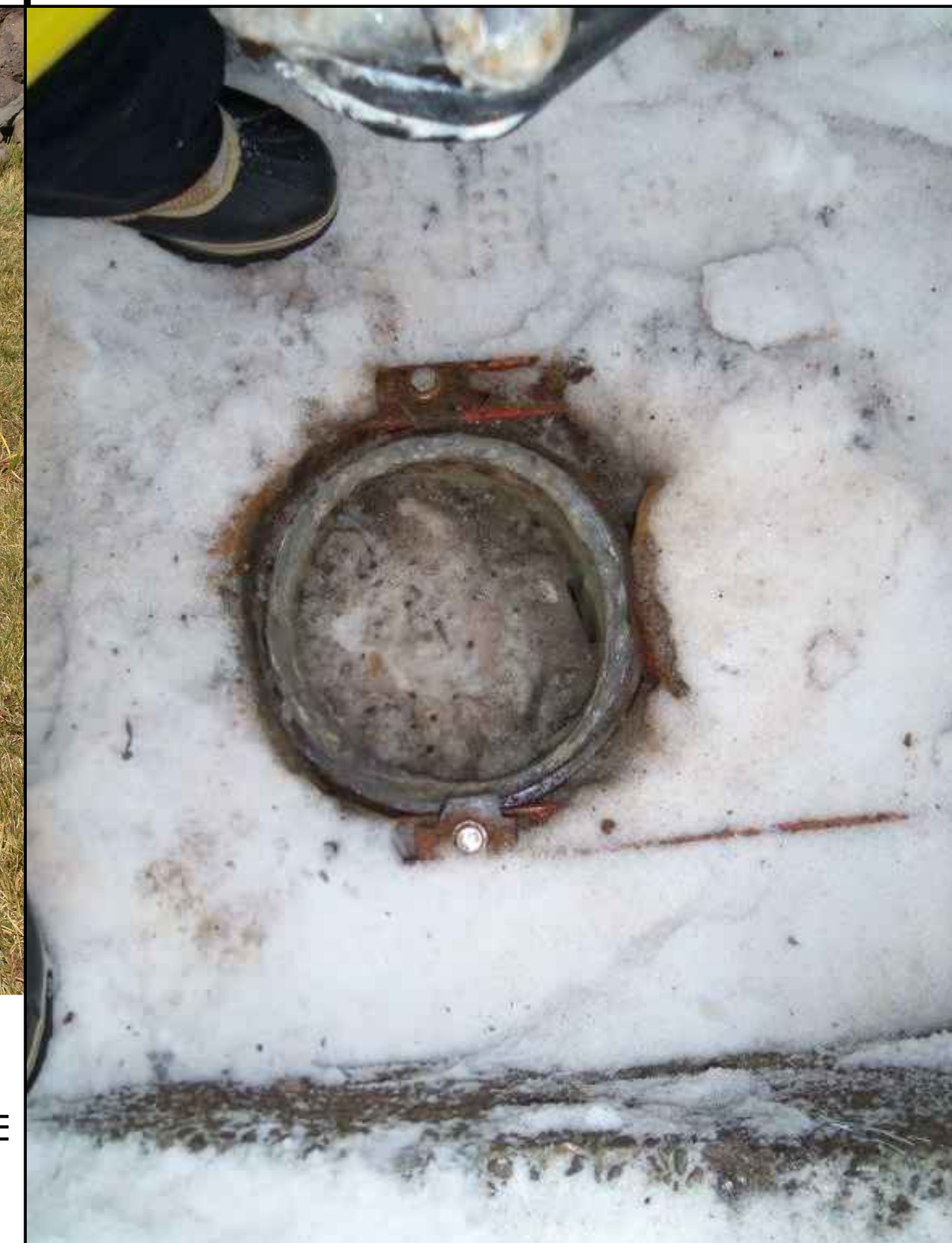
PHOTO 6: STEAM IS ADDED TO COMPRESSED AIR FROM A CONNECTION ON THE PIPE LINER AIR INVERSION TOOL (NOT SHOWN, BUT SHOWN IN PHOTO 5) TO ACTIVATE THE CATALYST CURING THE RESIN THEREBY COMPLETING THE CURED IN PIPE PROCESS FOR THE PROJECT
