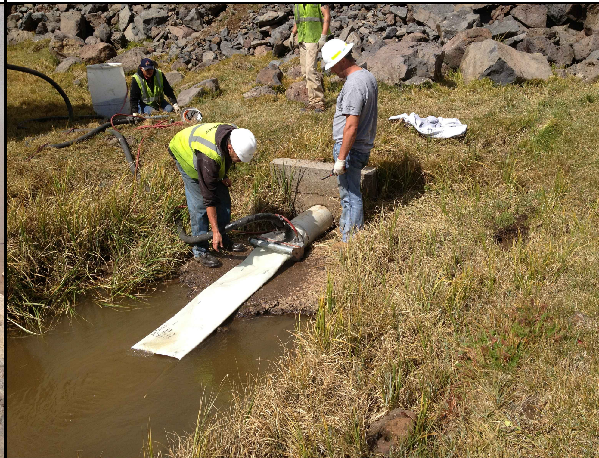
PHOTO 5: END OF INNER PORTION OF 2 PART LINER APPROACHING PIPE LINER AIR INVERSION TOOL AND PUSHED NEARLY ALL THE WAY BACK THROUGH THE OUTER LINER AND HOST PIPE TOWARD THE RESERVOIR SIDE. PHOTO AT THE OUTLET SIDE.
