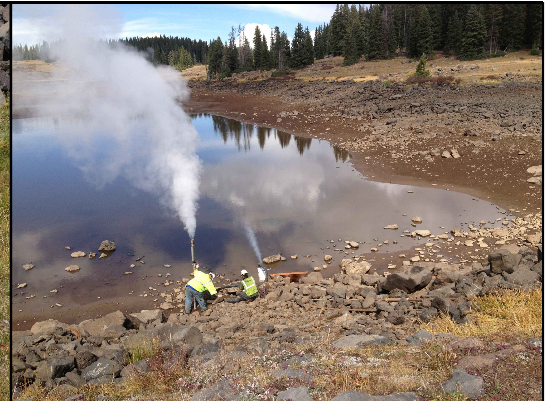
PHOTO 6: STEAM IS ADDED TO COMPRESSED AIR FROM A CONNECTION ON THE PIPE LINER AIR INVERSION TOOL (NOT SHOWN, BUT SHOWN IN PHOTO 5) TO ACTIVATE THE CATALYST CURING THE RESIN THEREBY COMPLETING THE CURED IN PIPE PROCESS FOR THE PROJECT
