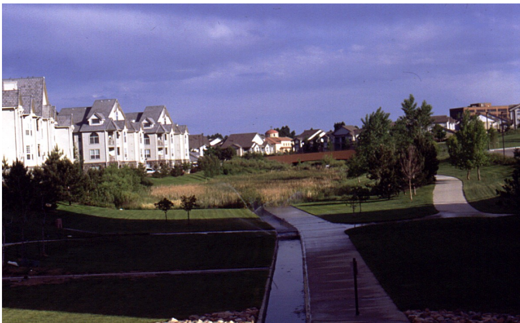
Private development oriented to open space
