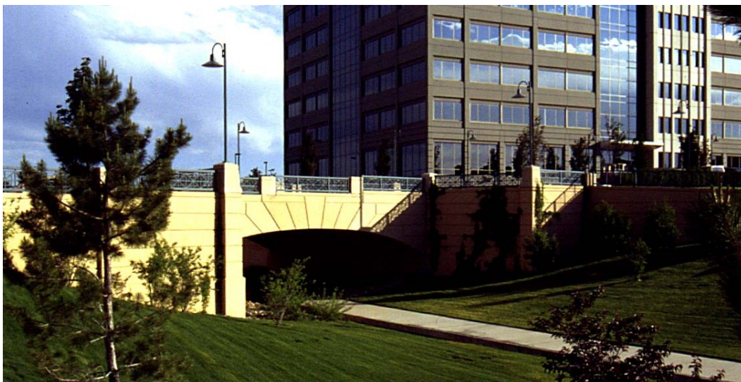
Open space incorporates drainage facility and amenities
