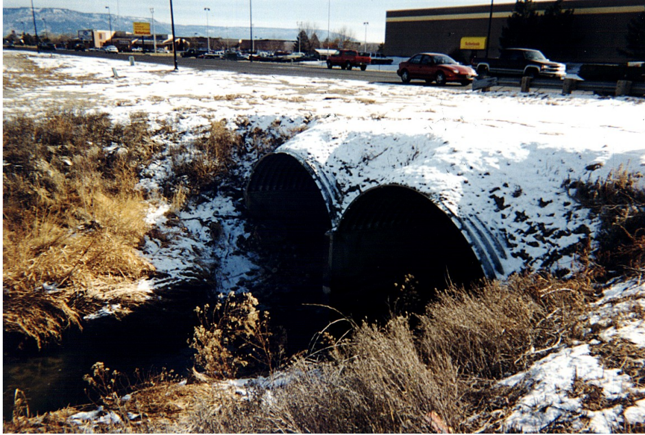
Existing Leach Creek drainage structure along 24 Road
