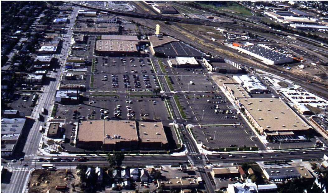
Buildings at the edges of project site with pedestrian connections through parking areas
