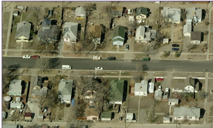
Existing Residential Subarea Streetscape Character
