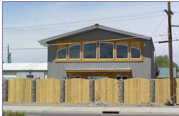
Screening Example on Riverside Parkway
