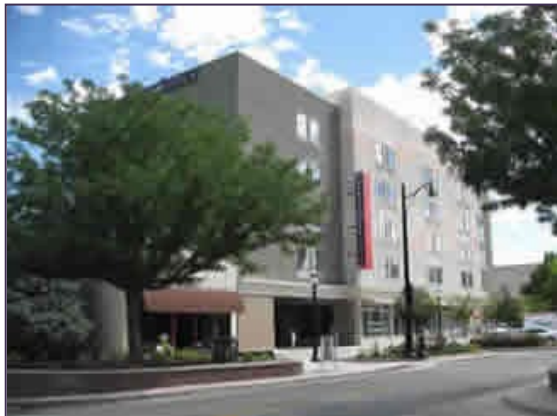
Existing Facades with Diminishing
